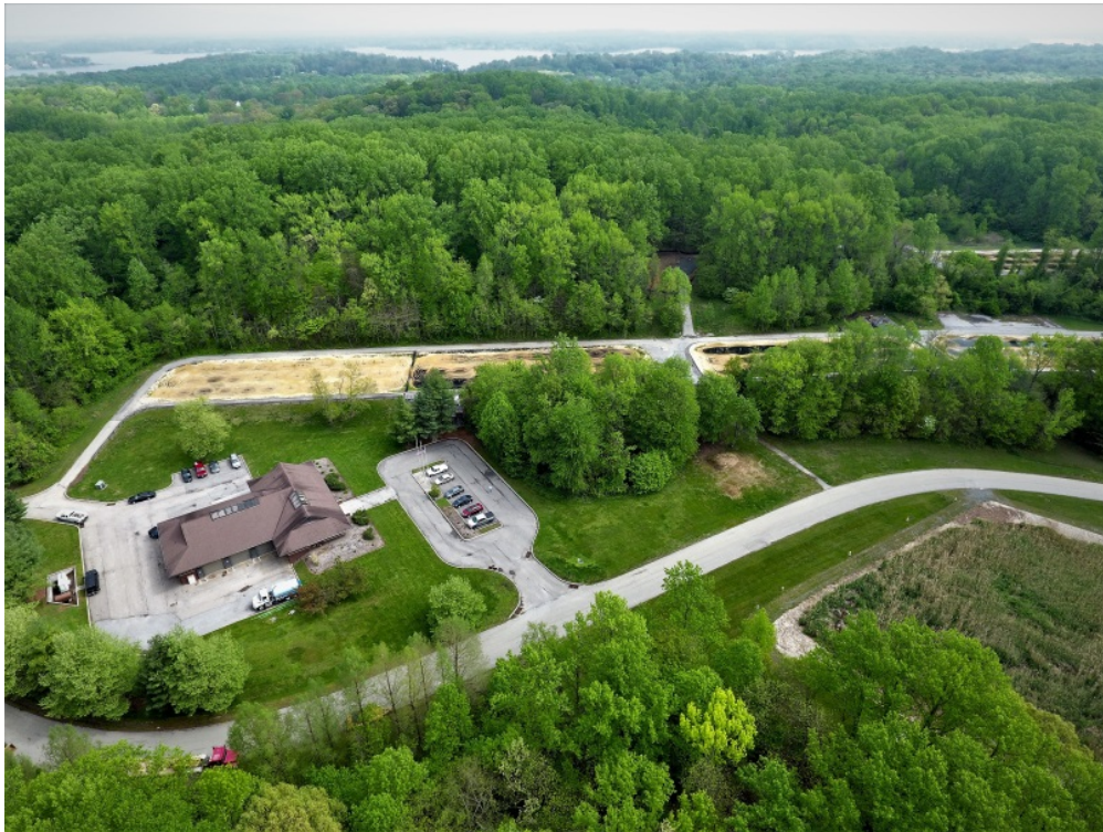
Existing operations building with parking & sand filters beyond
