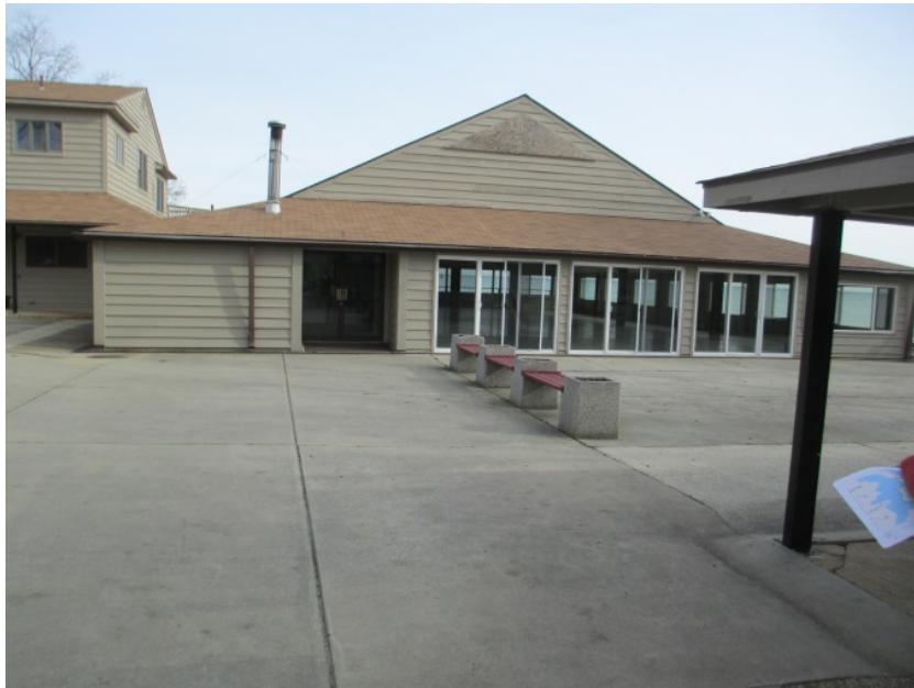
Existing Mayo Beach Event Building & Outdoor Patio
