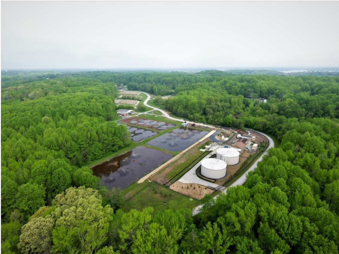
Existing peat filters and water tanks looking North up Pure Water Way
